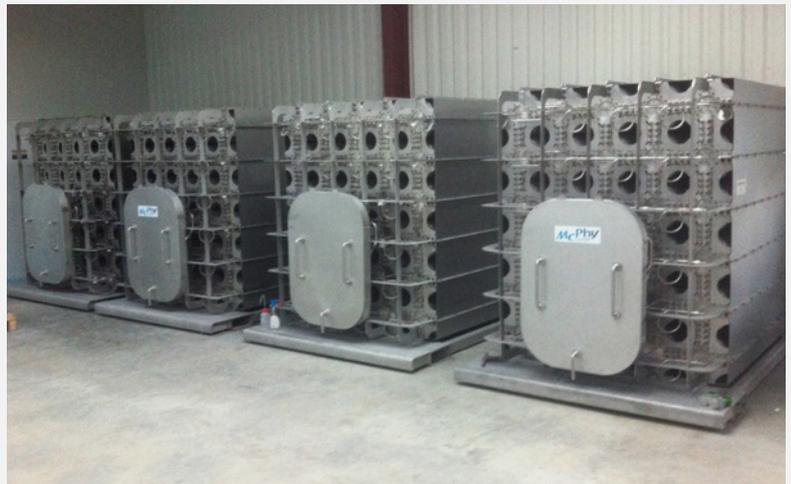
**Figure 1:** Four Hydrogen storage blocks containing 150 kg H<sub>2</sub> each (Source: McPhy Energy)
